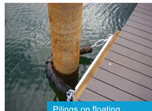
Pilings on floating walkway. McDonald Creek boat launch.
