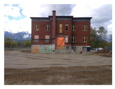
A small portion of foundation will remain to ensure the chimney is properly supported. Once repurposing of the building is confirmed, a decision can be made regarding the demolition of the chimney.
