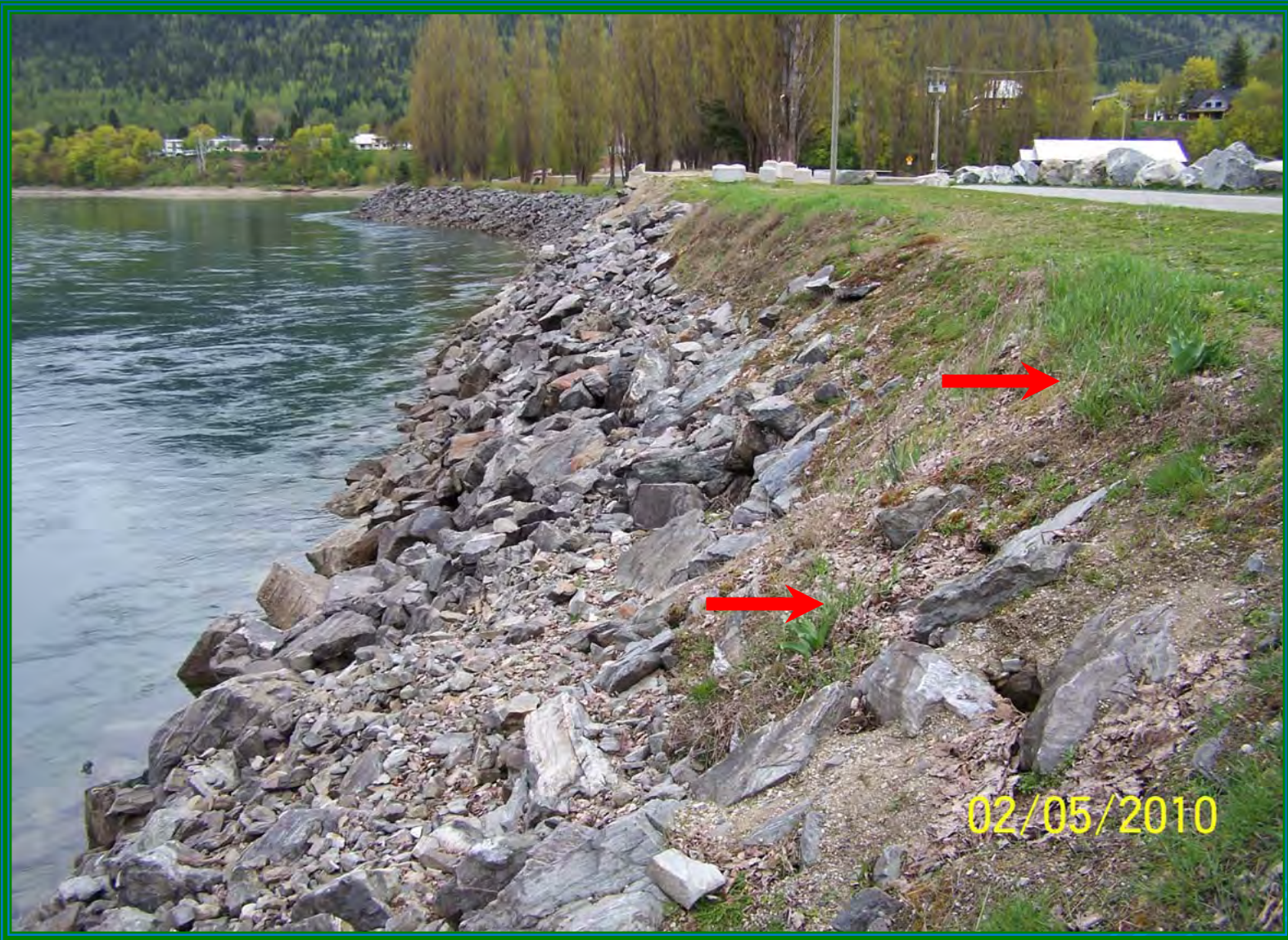
#7 : Incision Centennial Park as channel has deepened the rip-rap bank armouring has settled into the river channel.
