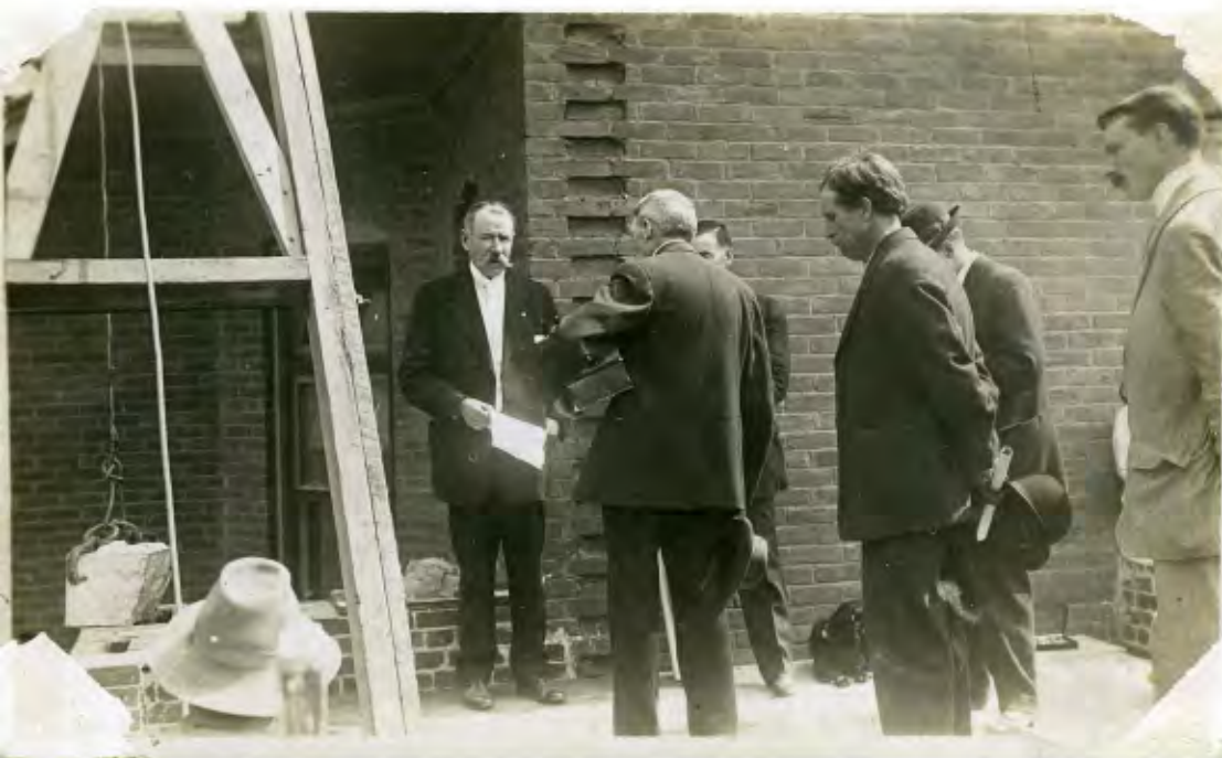
On August 21, 1912 the cornerstone was laid for the new brick Queen Victoria Hospital. MLA Thomas Taylor is facing the camera.
