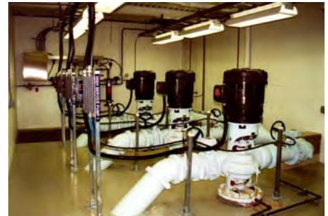
Greeley Creek Filtration Plant
