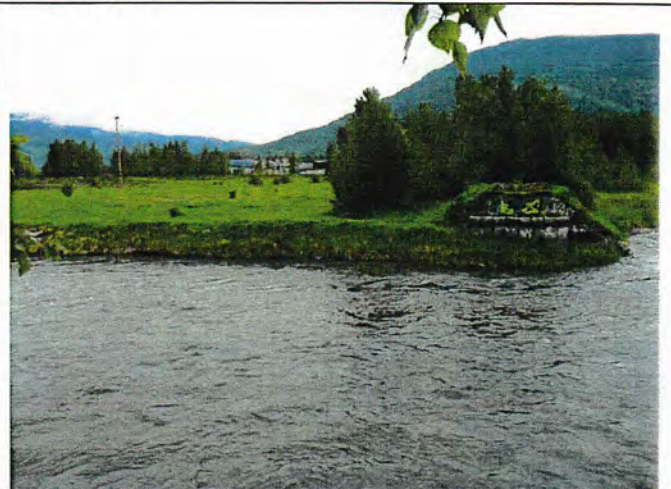
View north to north bridge abutment from the south abutment.
