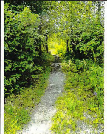
Last section of old RR grade leading to old bridge abutment in distance.
