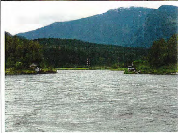
View west of N & S side of bridge abutments of old RR Bridge over the Illecillewaet River.
