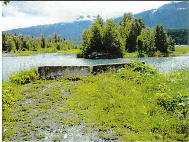
View from north bridge abutment to the south bridge abutment.
